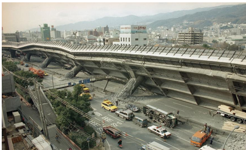
Figura 6.5. Autopista elevada de Kobe colapsada tras el terremoto. Nota. De Have we learned enough from the 1995 Kobe quake? , por The Japan Times, 2020. Have we learned enough from the 1995 Kobe quake? - The Japan Times
