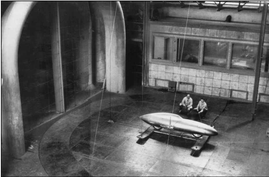
The NSU record breaker being tested in the full size wind tunnel at the Stuttgart Technical College. The size of such installations is quite apparent from this photograph. Compare this to the much smaller tunnel used by the author to test the 1/6 th scale model of the QL, pictured earlier.
