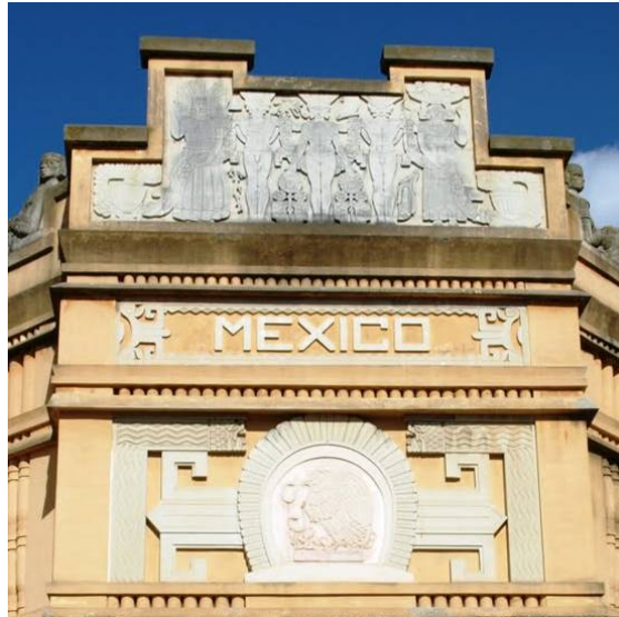
Foto 184. Remate fachada principal
