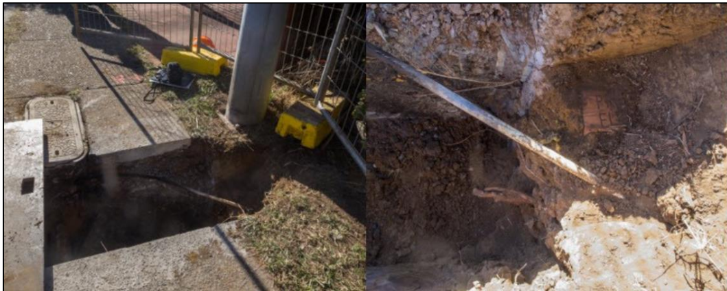
Figure 1: Trench excavation site where works were being undertaken [20]
