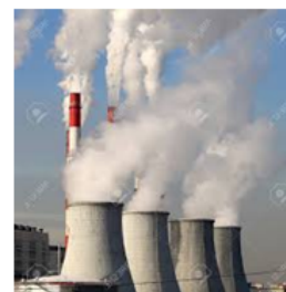
Coal burning power plant
