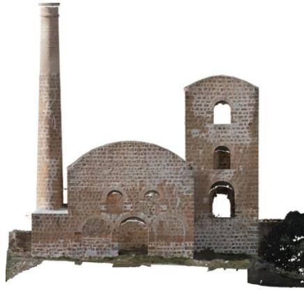
Image 1. – Santa Annie – view of east facade from Metashape, Linares, Spain Source: Author's archive
