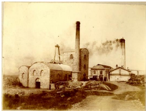
Image 10. - Engine and boiler houses in La Tortilla mines at the beginning of twentieth century
