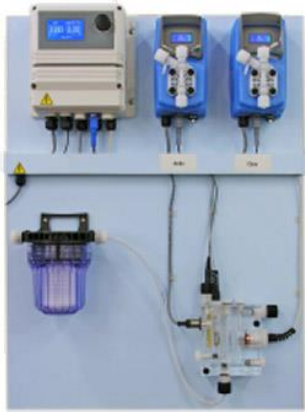
Fig. 4-45 Panel cloro libre – pH LDPHCL/6 [33]
