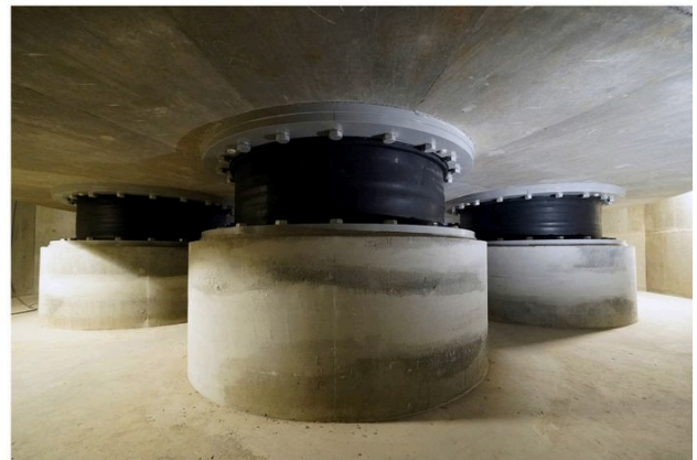
Tokyo Skytree is designed to let strong wind pass through the gaps between trusses. At its base, rubber dampers are used to reduce movement. Photographer: Toru Hanai/Bloomberg
