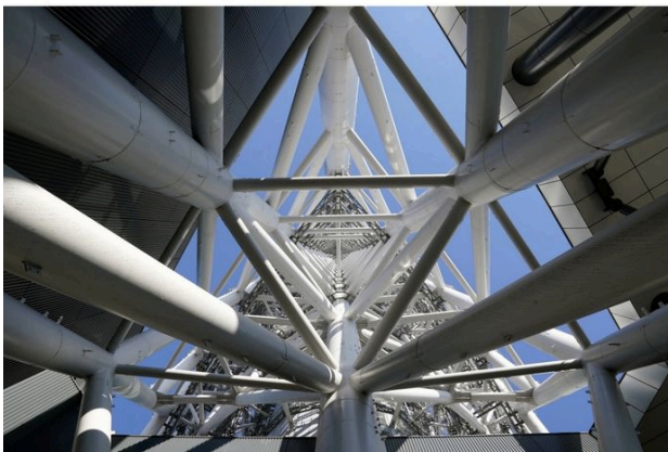
Tokyo Skytree is designed to let strong wind pass through the gaps between trusses. At its base, rubber dampers are used to reduce movement. Photographer: Toru Hanai/Bloomberg
